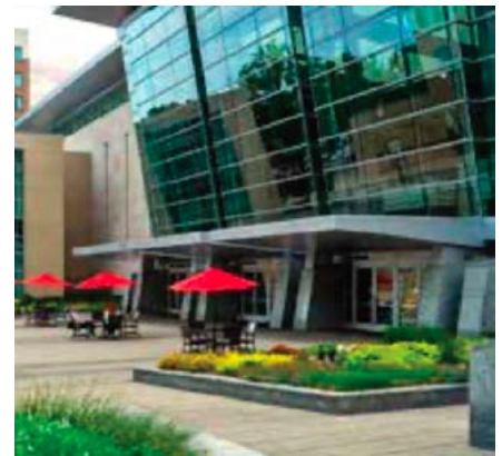
Drop-off zone in front of the building
